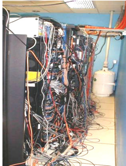
Figure 3 – Example of unstructured cabling
